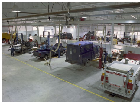
Interior Vehicle Area of Fleet Building
