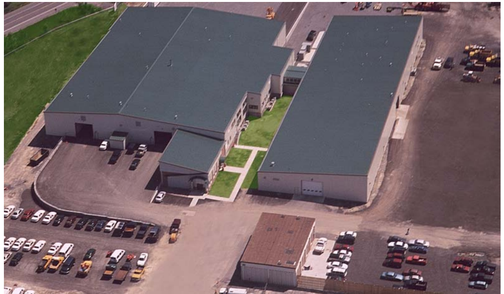
Aerial View of Completed Fleet Center
